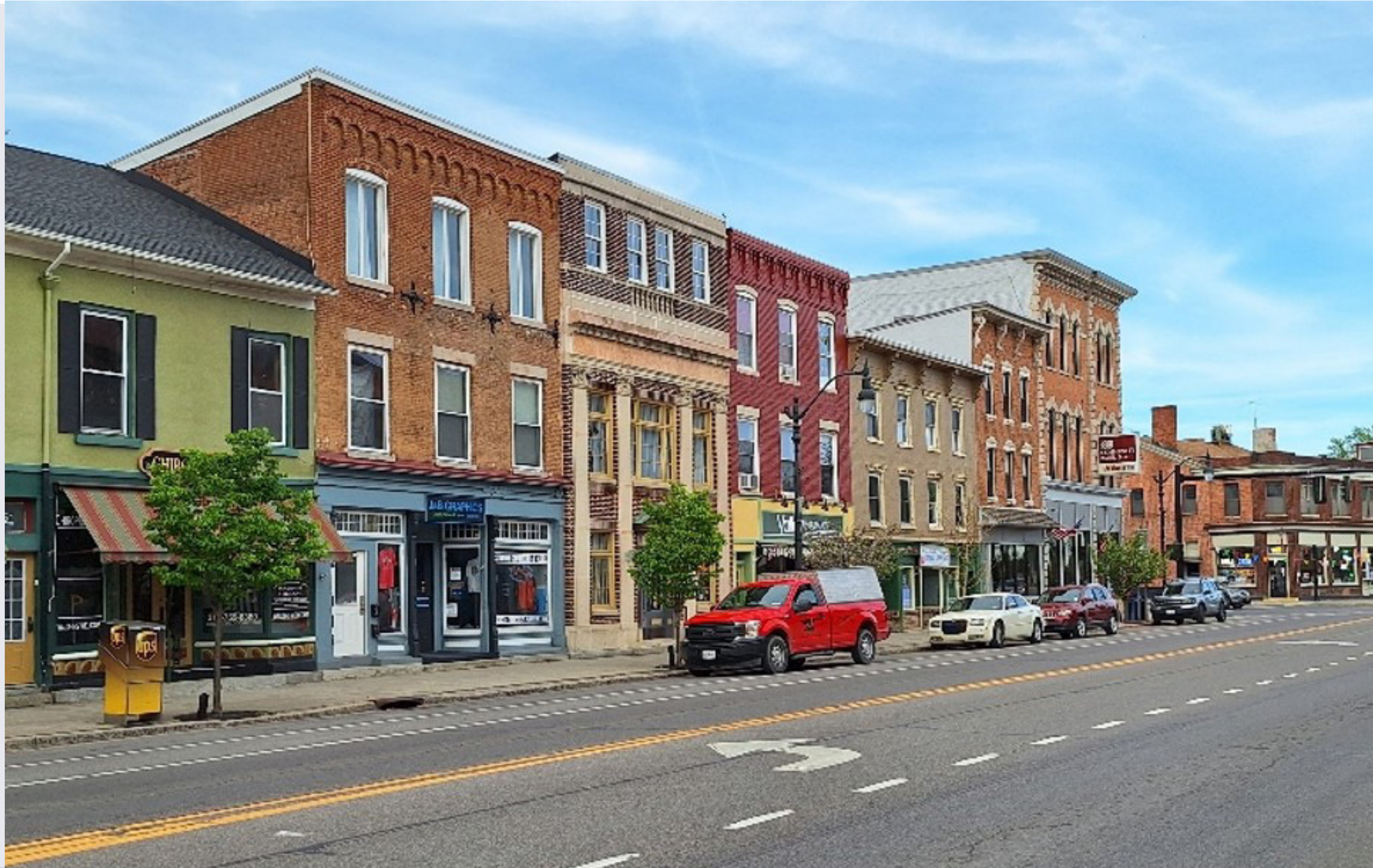
Intact, historic building fabric along Main Street
